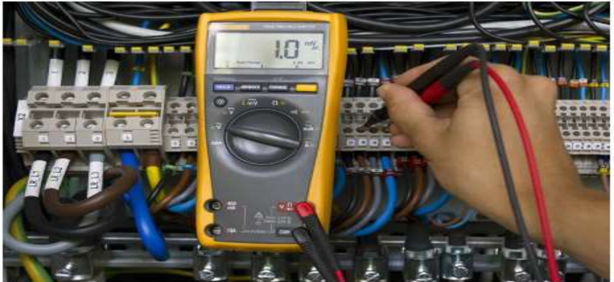
Figure 118: Testing a control board using instrument
