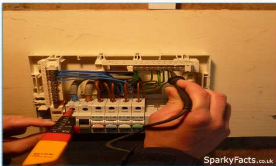
Figure 314 Test between Neutral and Earth terminals
