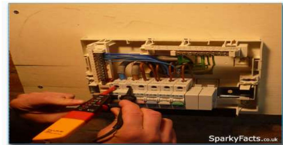
Figure 312 Test between Line and Neutral terminals
